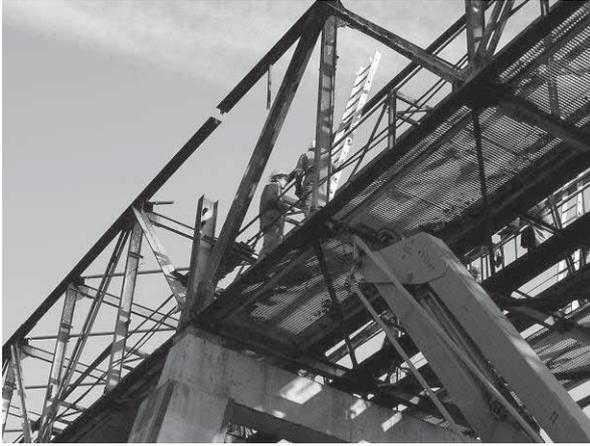
Figure 4.1.7. Replacing of the end frame.
