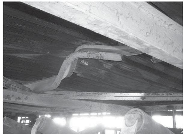
Figure 4.1.6. Deformed purlins.
