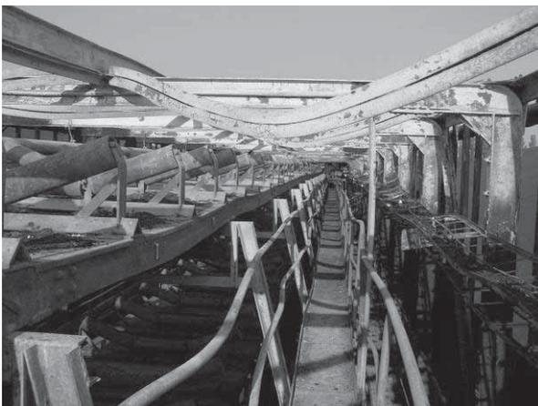
Figure 4.1.5. Deformed upper stiffening truss.
